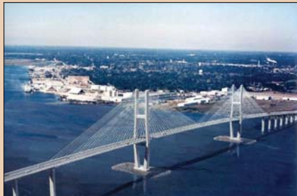
Sidney Lanier Bridge Brunswick, GA
