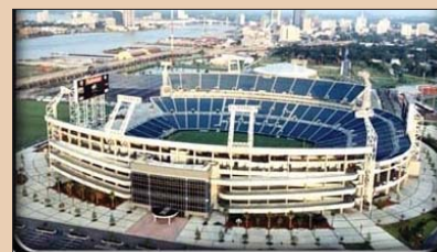
Jaguar Stadium Jacksonville, FL
